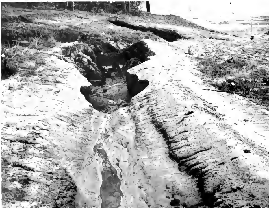
Intercepting drain ditches at top of slope like above also need vegetative protection
